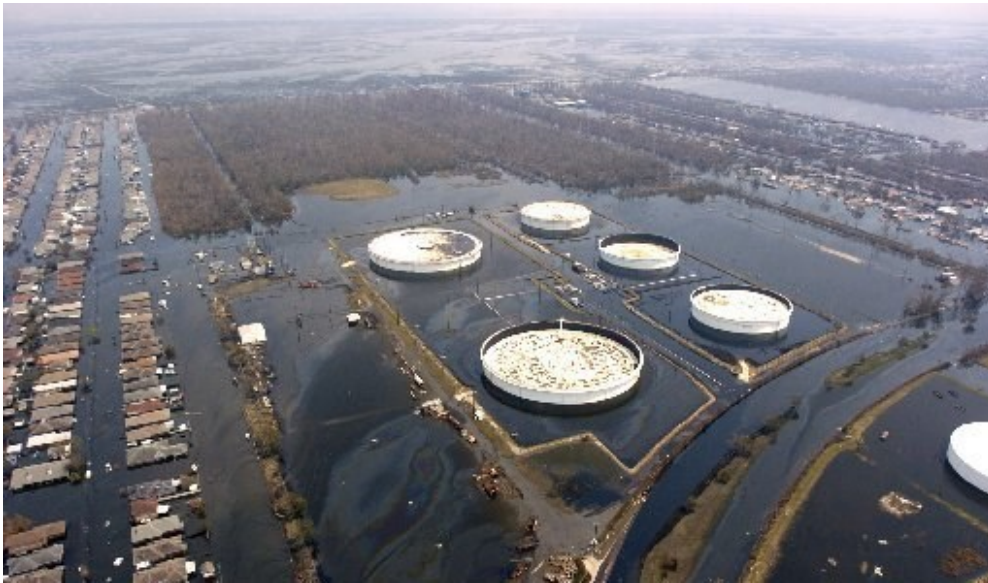
Figure 1. The Murphy Oil facility near New Orleans was flooded by Hurricane Katrina, releasing about 1 million gallons of crude oil from a storage tank that was lifted from its foundation.
