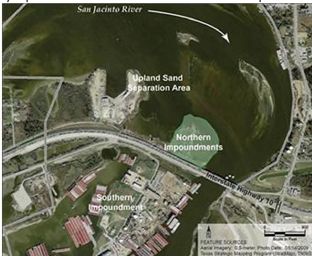
Figure 5. Graphic showing the location of the San Jacinto Pits both north and south of IH-10 where it crosses the San Jacinto River.
